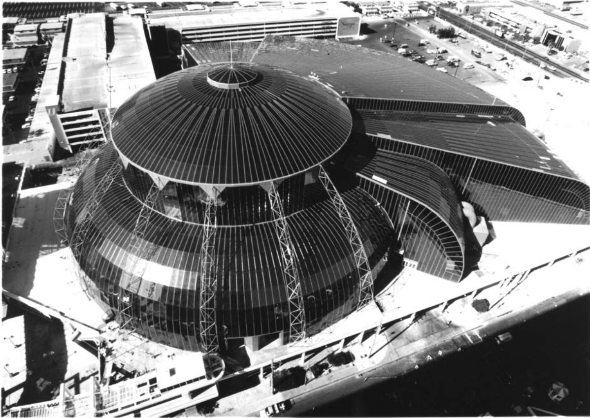
FIG. 5 Sloped SSG System
