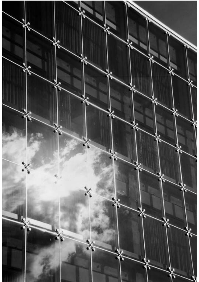
FIG. 4 Four-Side SSG System
