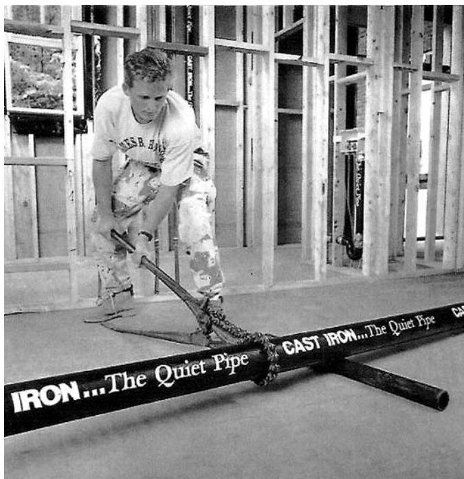
FIG. X1.1 Snap Cutter
