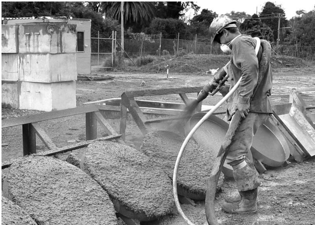
FIG. X1.5 Manual Spraying of Panels
