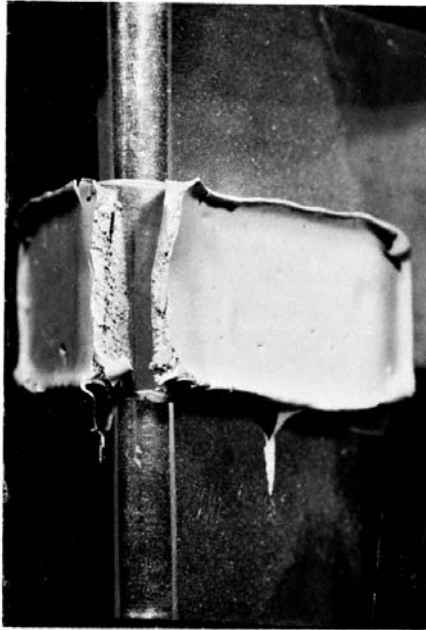
(a) Complete Cracking and Adhesive Failure
