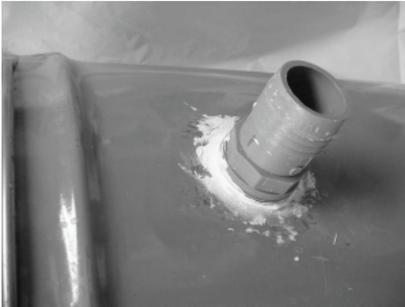
FIG. A1.5 Overflow Tube Detail
